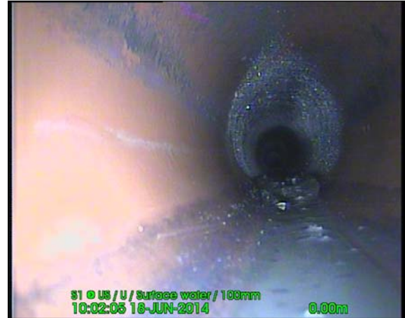
Photo: 140618_1002A-Survey.jpg 0m, Water level 5 % of the vertical dimension
