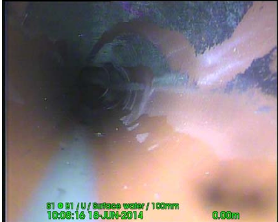
Photo: 140618_1008C-Survey.jpg 0m, Start node type, manhole reference number: S1
