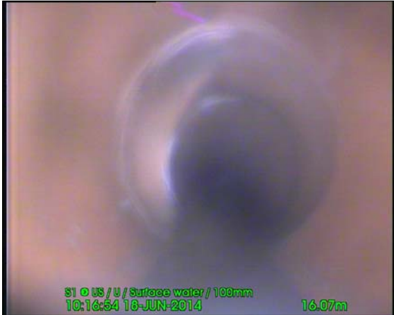
Photo: 140618_1016B-Survey.jpg 16.07m, Junction from 9 O'Clock diameter: 100 mm
