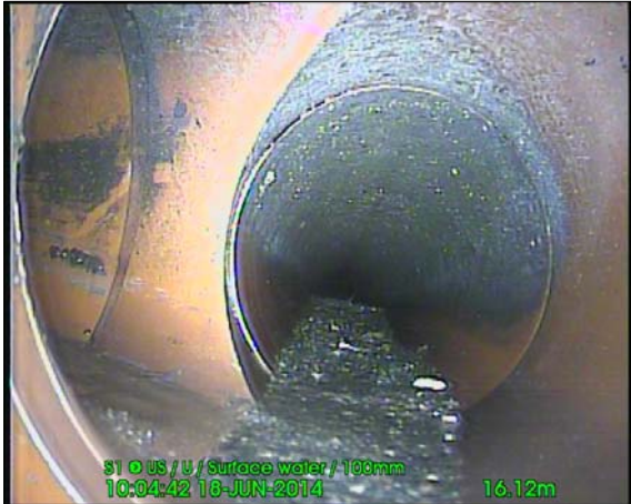
Photo: 140618_1004B-Survey.jpg 16.12m, Junction from 9 O'Clock diameter: 100 mm
