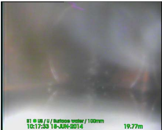
Photo: 140618_1017B-Survey.jpg 19.77m, Junction from 3 O'Clock diameter: 100 mm
