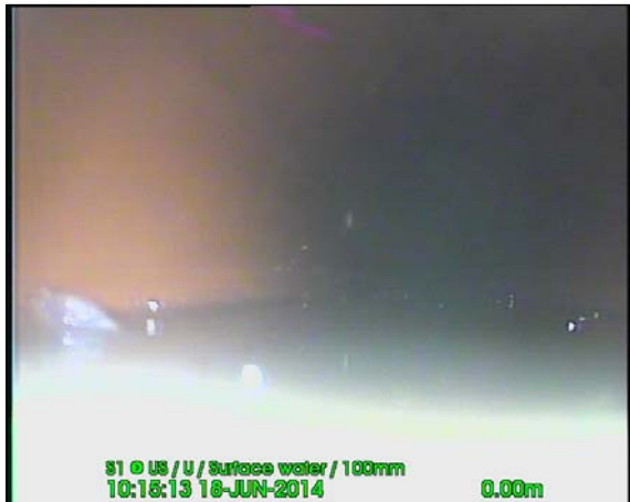
Photo: 140618_1015C-Survey.jpg 0m, Start node type, manhole reference number: S1
