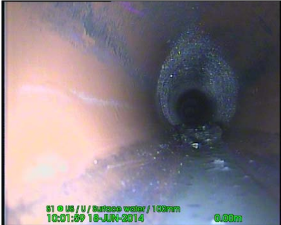
Photo: 140618_1001C-Survey.jpg 0m, Start node type, manhole reference number: S1
